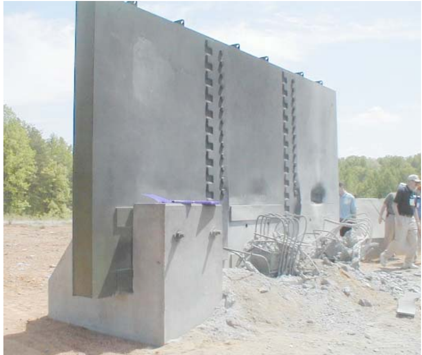
Figure 2 – Since the TNT charge decimated the concrete bolster on which it was sitting, the TNT charge was placed on a different bolster each day. This photograph was taken after the second day. The bolster to be used on the third day can be seen in the foreground. (The charge will be placed where the blue folder in the photograph is located.) The remnants of the bolsters used on the first and second day can be seen along the center and right side of the wall. The rebar in the bolsters is #7. Damage to the blast wall itself can also be observed behind the sites of the first and second charges.
