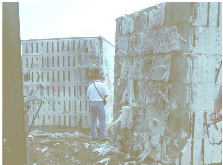
Figure 5 – Specimens D (left) and E (right). Specimen E had the closest standoff distance to the charge. The EPS was severely damaged, but the concrete maintained its structural integrity.
